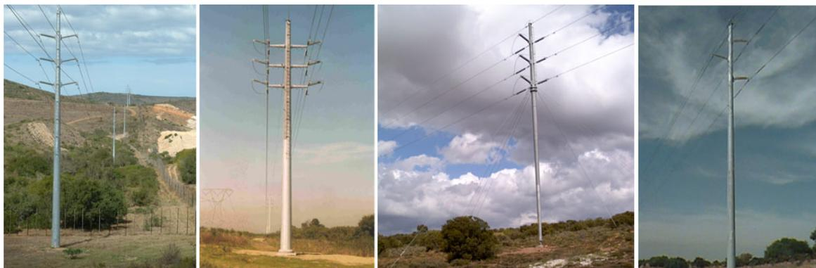
**Figure 7.10:** Examples of monopole distribution power line towers. Similar structures have been used for 400kV towers where space is limited
